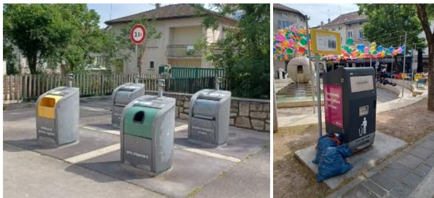
FIGURE 91 : CONTENEURS ENTERRES A BOURG-EN-BRESSE (SOURCE : EVEN CONSEIL)
